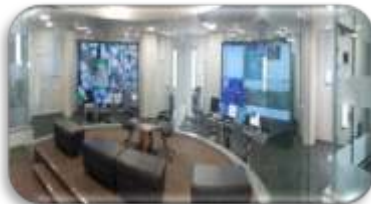
Smart Infrastructure - City Command & Control Centre (C4)
