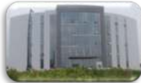
Tier IV Data Centre - 900 Racks
