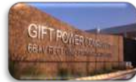
Dual power supply at Power Station with building level Back-up power facility
