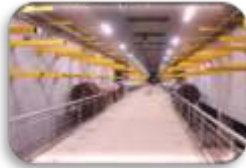
Underground Utility Tunnel
